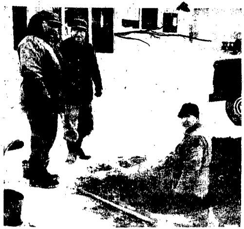
BELOW ZERO weather or not, these three Dixon men had to get to a water main break and dug into Main street to get to it. Left to right are Jim Saunders, Claire Gleason and Lloyd Matson.
